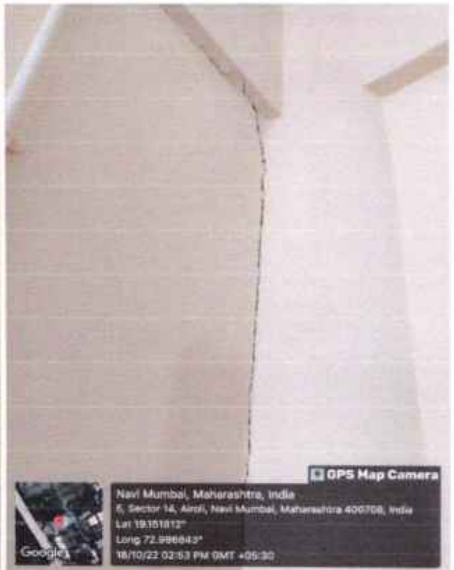
Cracks and Seepage
